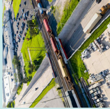
CREATE GS14 Structural Engineer
