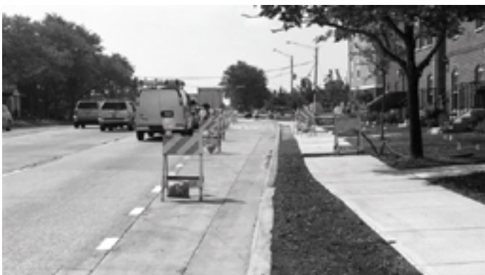
Figure 11. The intersection improvements at Roselle Road and Schaumburg Road provide new turn lanes to reduce congestion at this busy intersection, along with new sidewalks, curbs and gutters.
