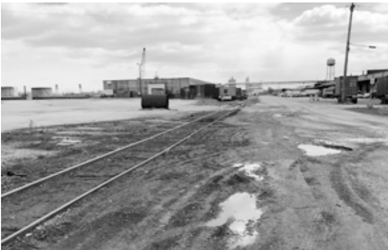
Figure 5. While just 1.16 miles in length, the Butler Drive corridor services 13 companies, which employ 150 full-time employees and 22 part-time employees. Collectively, businesses served by Butler Drive generate freight volumes equating to 830 trucks, 75 rail cars and four barges on a weekly basis. This level of traffic, combined with deferred maintenance, has resulted in poor pavement quality and Butler Drive is unpaved along the western portion of the corridor.
