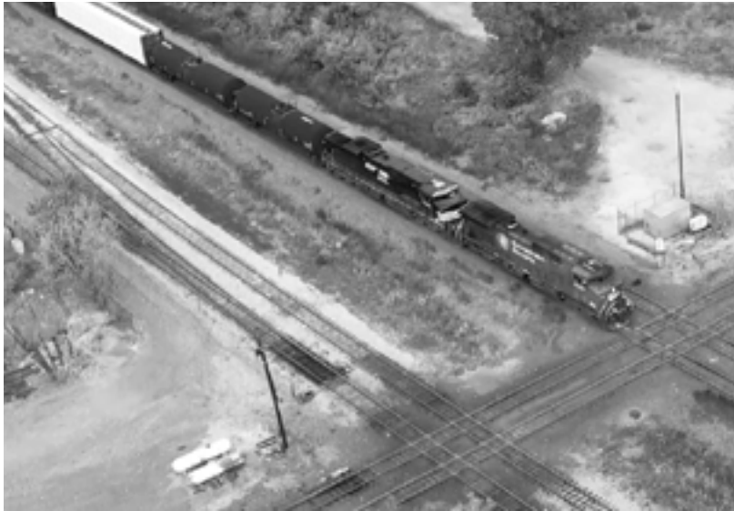
Figure 3. The 75th Street Corridor Improvement Project is the single largest project remaining in the CREATE program, and will address major rail bottlenecks. At this location, the north-south rail lines will be separated from the east-west rail lines, eliminating a major point of congestion.
