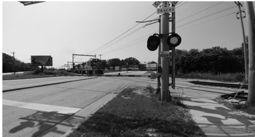
Figure 4: The Burnham Multimodal Connector over CSX and NICTD railways will help close a gap in the regional trail network and will increase safety for pedestrians and cyclists by providing an alternative crossing at this junction.
